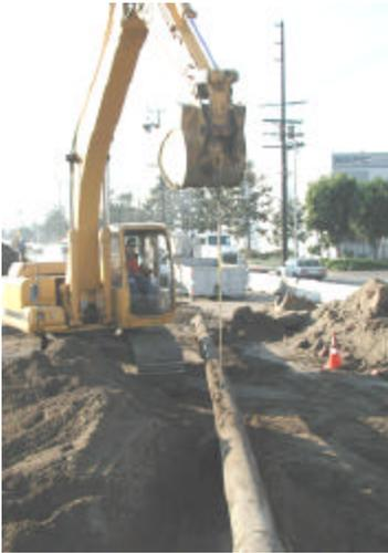
NRCES excavates contaminated soil and pipeline on the Alameda Corridor in Los Angeles, CA
